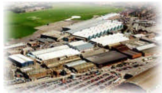
Westland Helicopters Ltd facilities in Yeovil, England
